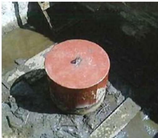
**Figure 3a: Abandoned well with steel plate**
